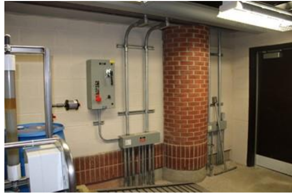
Plate 18: Exterior bricks located within main WWTP building
