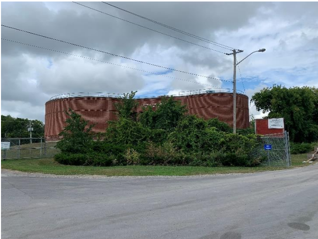
Photo 11: Site conditions of Wastewater Treatment Plant (Site 3). Facing West.
