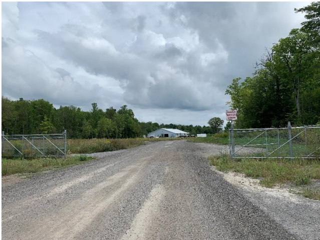
Photo 5: Site conditions of Water Reservoir Site (Site 2). Facing East.
