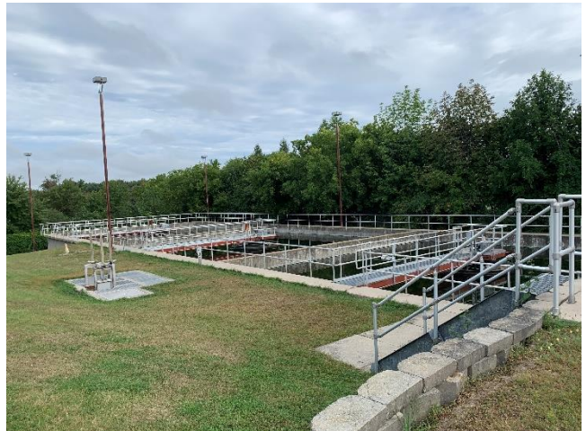
Photo 12: Site conditions of Site 3. Facing Northeast.
