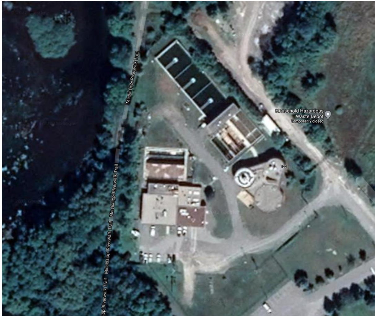
Figure 3.9: Carleton Place WWTP Aerial View
